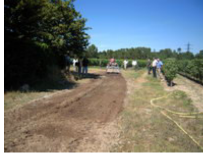
Work done with ROCAMIX
